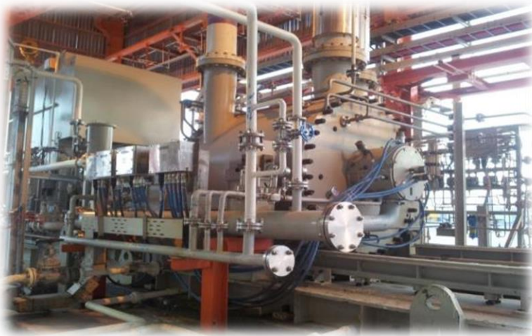
Propane Refrigeration Compressor EBS45-2+3 for South Pars Fields, Iran
